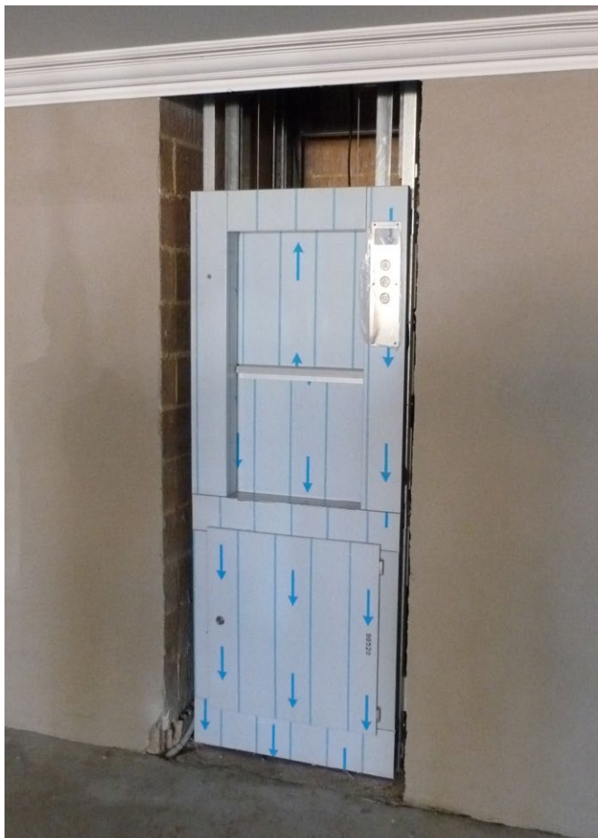
Ground floor in garage.
