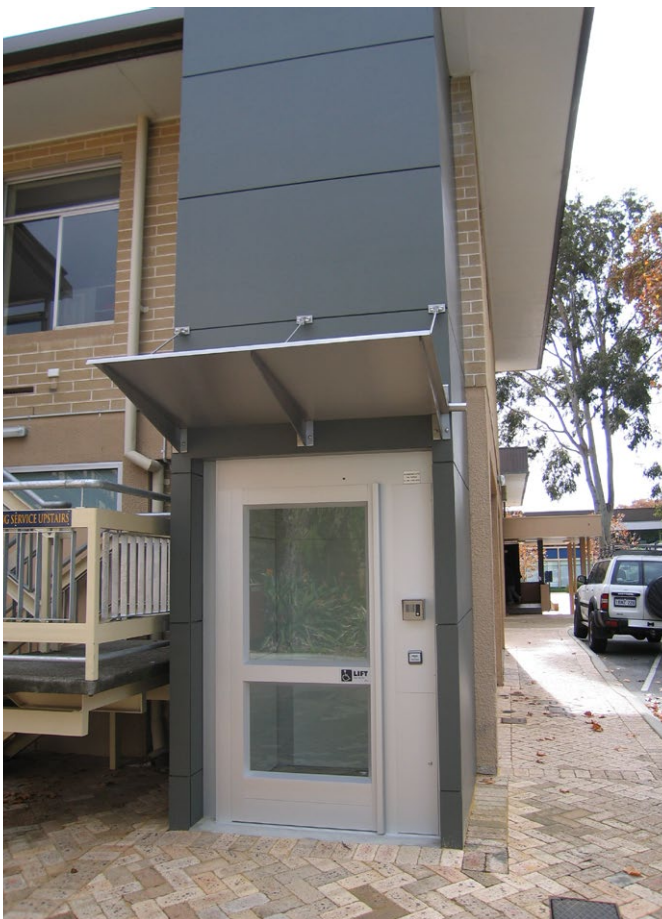
Existing building - Christchurch Grammar:
