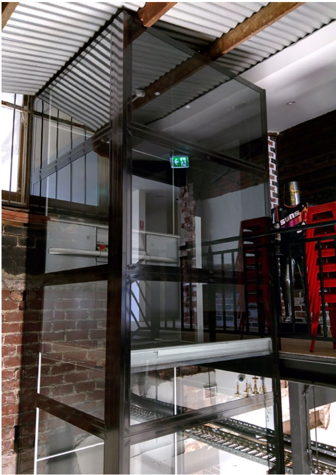
A5000 Glass Shaft - Eight Avenue, Maylands:
