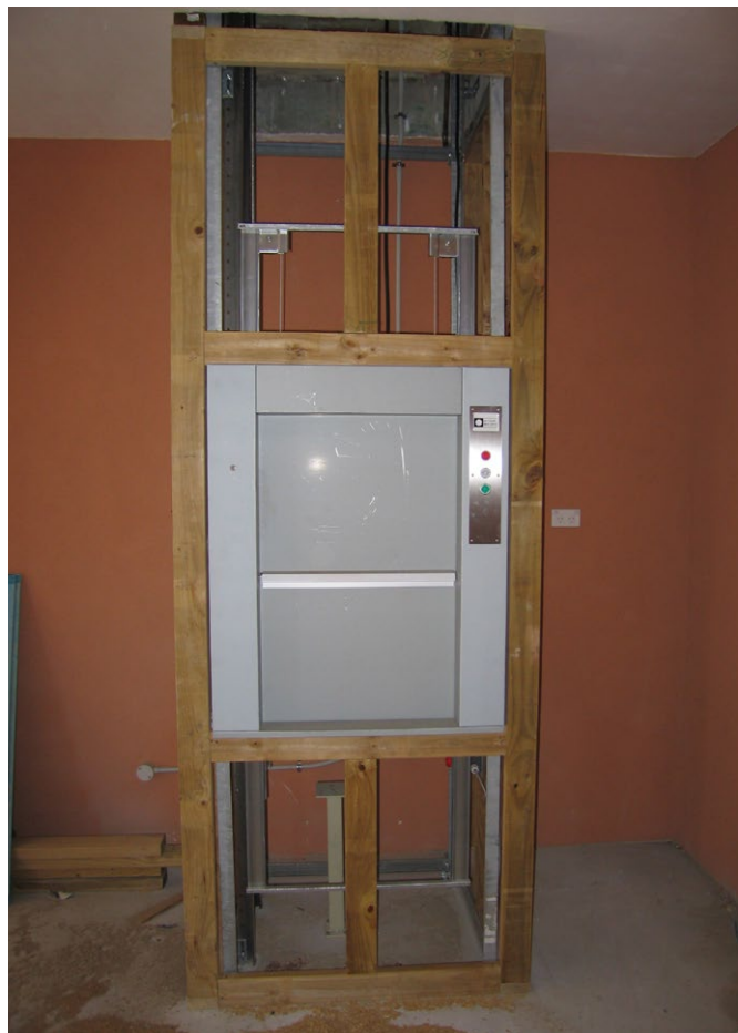
Self-supporting frame with stud wall surround.
